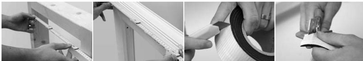
Remove approx. 20 cm of the covering paper. Adhere the tape to the frame leaving an excess length (lower joint width dimension).
