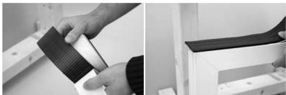
Cut off the tape at the upper edge leaving an excess length and form a butt joint in the corner so that it is flush with the outer edge of the frame. When reaching the end of the roll, form a butt joint and cut off the last and first 2cm. If necessary, fill in cross joints/breakouts with a suitable sealing compound (e.g. MS-polymer).
